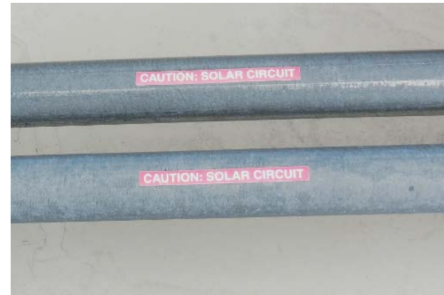
Examples of PV system marking
